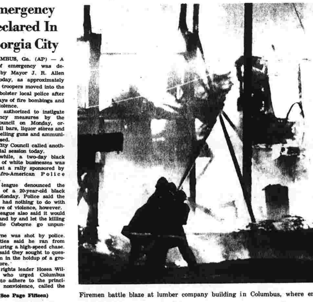
Firemen battle blaze at lumber company building in Columbus, where emergency state was declared. (AP photo)
